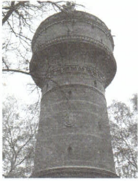
Opole Water Tower
